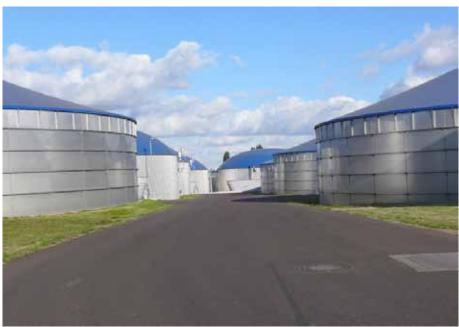
At the plant in Arneburg, about 6 million cubic metres of biomethane will be produced every year in four fermenters and six digestate storage units.
